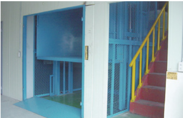
▲ 1층모습-TWO MAST Type
